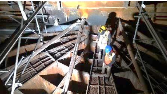
RAPH basket replacement work U/P
