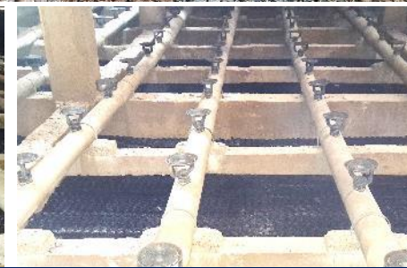
New CT Fills (after replacement) & new water distribution channel with spray nozzles
