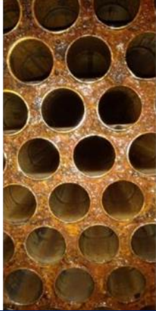
Condenser tubes after cleaning
