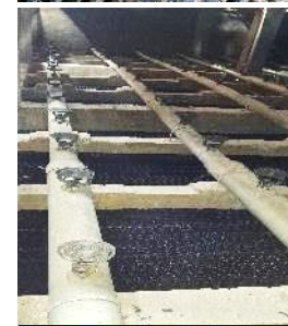
New CT Fills (after replacement) & new water distribution channel with spray nozzles
